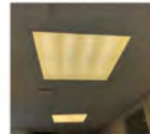
• First Floor Corridor • Before
