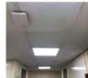
• First Floor Corridor • After
